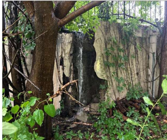
Exterior wall of parking structure with flowing water
